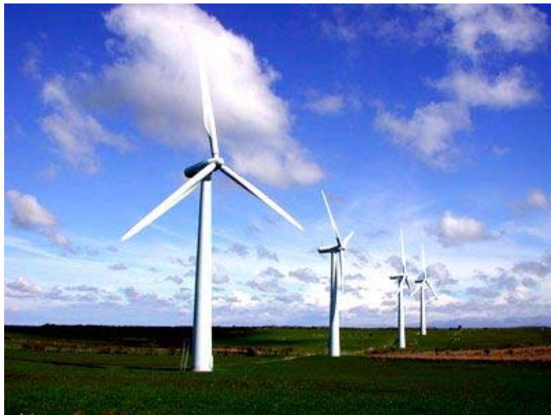
Figure 1: Typical wind turbines
