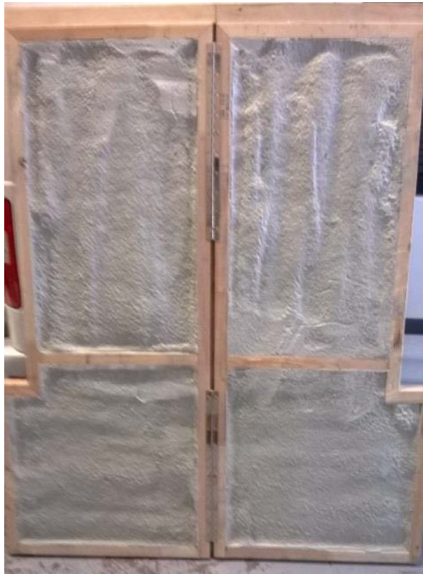
Figure 4.19. Floor panel after being insulated with closed-cell PU foam
