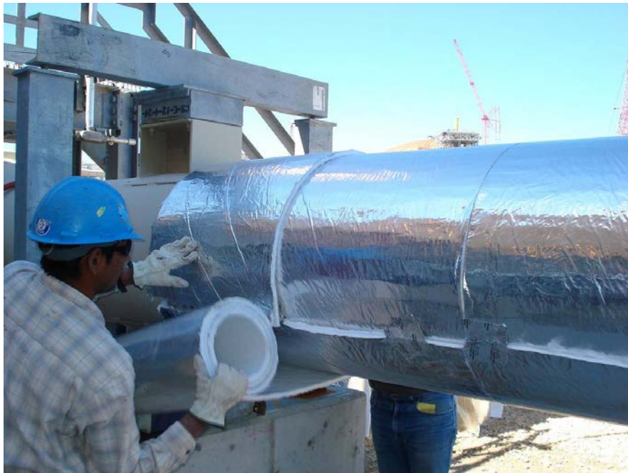
Figure 2.14. Flexible industrial aerogel blanket with integral vapour barrier for sub-ambient and cryogenic applications [37]
