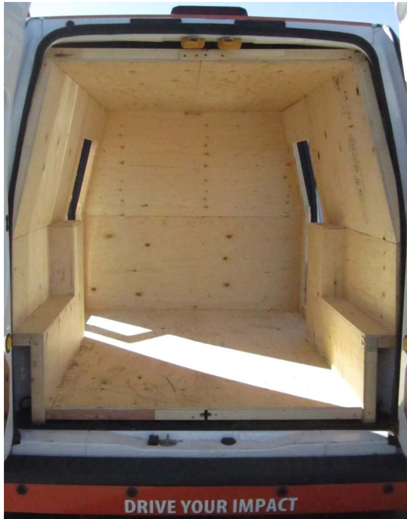
Figure 4.18. Final assembly of wooden panels inside the Ford transit van
