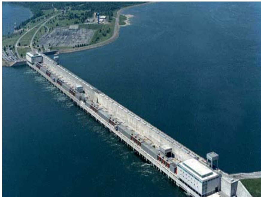
Figure 1. Canada/USA Border on Dam.
