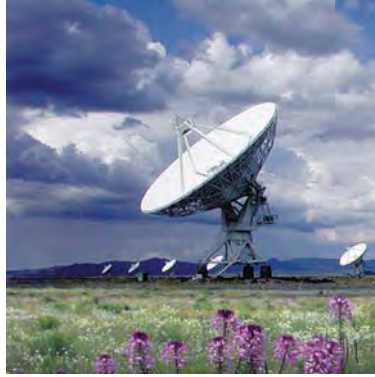
FIGURE 33-36 The very large array (VLA) of radio antennas is located near Socorro, New Mexico. The 25-m-diameter antennas are mounted on rails, which can be arranged in several configurations, and can be extended over a diameter of 36 km. The data from the antennas are combined electronically, so the array is really a single high-resolution telescope. (Courtesy of National Radio Astronomy Observatory/Associated Universities, Inc./National Science Foundation. Photographer: Kelly Gatlin. Digital composite: Patricia Smiley.)
