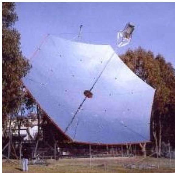
Fig. 9. The SG3 Big Dish prototype was built in Australia in 1994 and is the world's largest solar dish for generating electrical power, with an average diameter of roughly 23 m. It achieves a solar concentration of 1500 suns, and heats water in the range 400 °C–700 °C at 4.2–6.8 MPa. It has a design output of 320 kW. Source: Australian National University (ANU).
