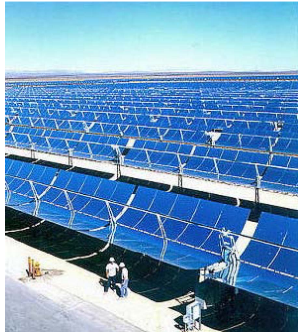
Fig. 3. The Solar Energy Generating Systems (SEGS) solar trough farm at Kramer Junction, California. The concept is that the reflective troughs focus sunlight on a pipe containing oil in a closed-cycle, which heats water to create steam to turbines. In total there are nine SEGS farms, with two at Dagett, five at Kramer Junction, and two at Harper Lake; all in California's Mojave Desert. The total area occupied is 2.4 sq km, generating 354 MW of power. These figures scale up to a footprint of 320 km by 320 km, if we were to supply 15 TW with this method. The nine plants have gradually been installed from 1984 to 1990, demonstrating over 20 years of performance without malfunction. Source: Power Corp.
