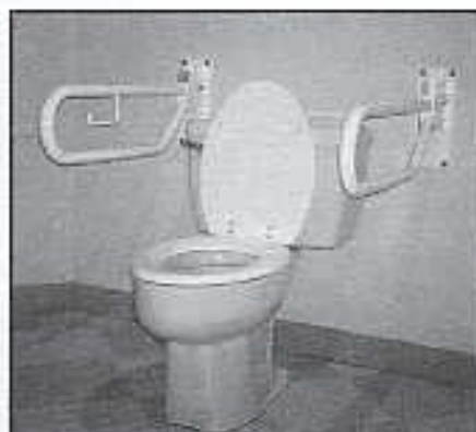
Toilet on angled wall
