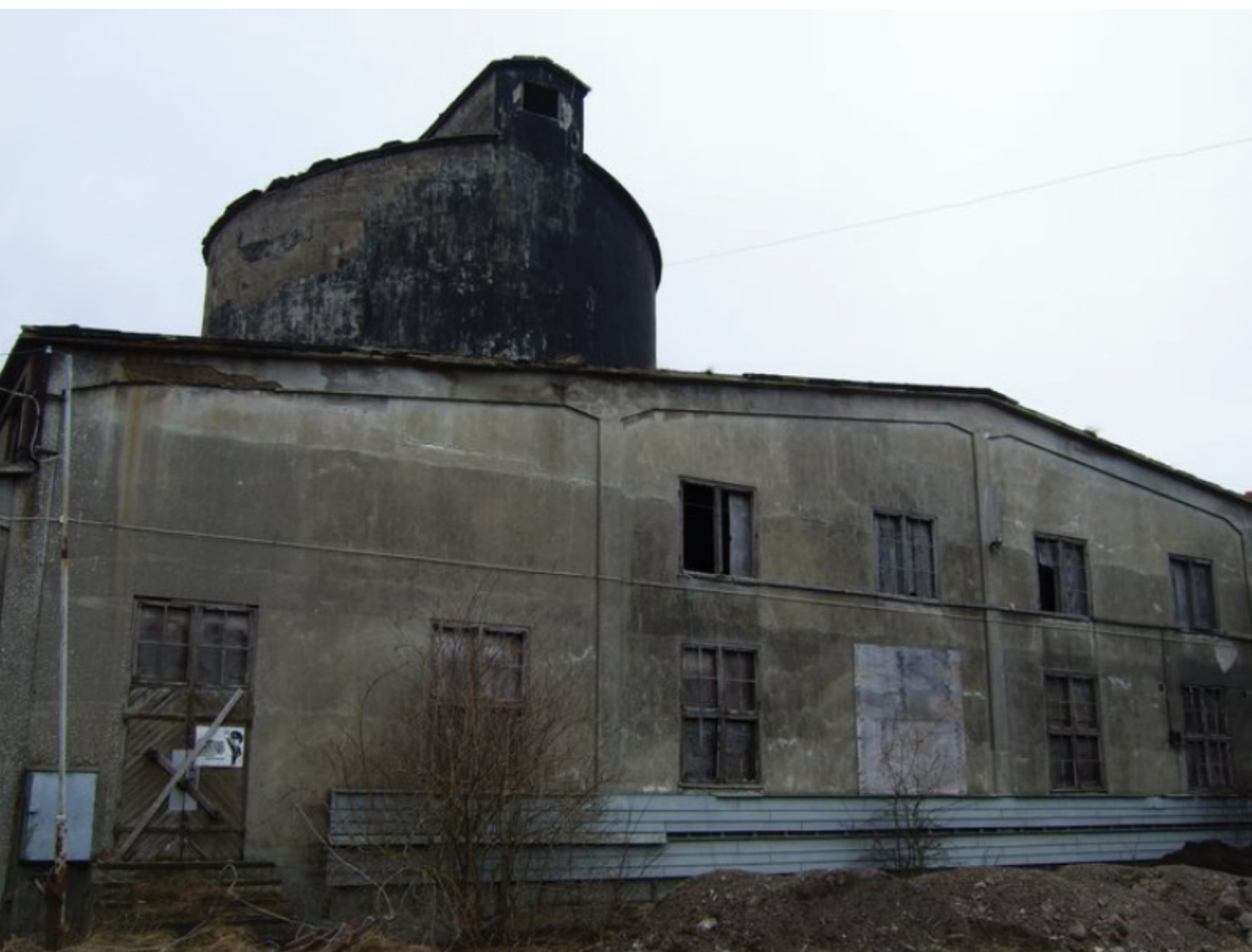
old derelict steel mill
