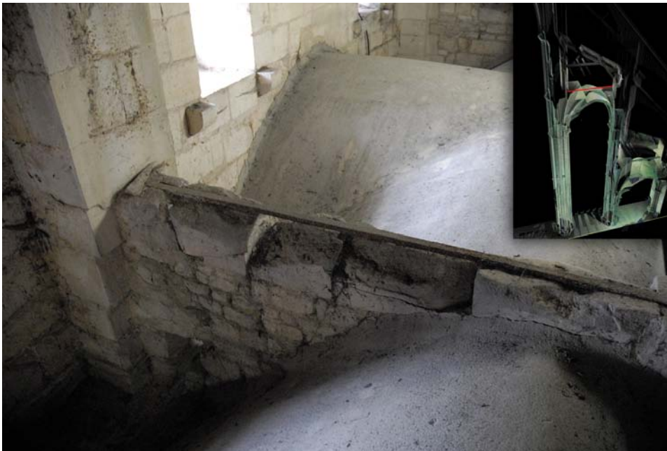
Figure 14 Bourges, Cathedral of Saint-Étienne. Iron tie over the inner aisle vaults with position indicated in the inset (photograph and laser image by author)
