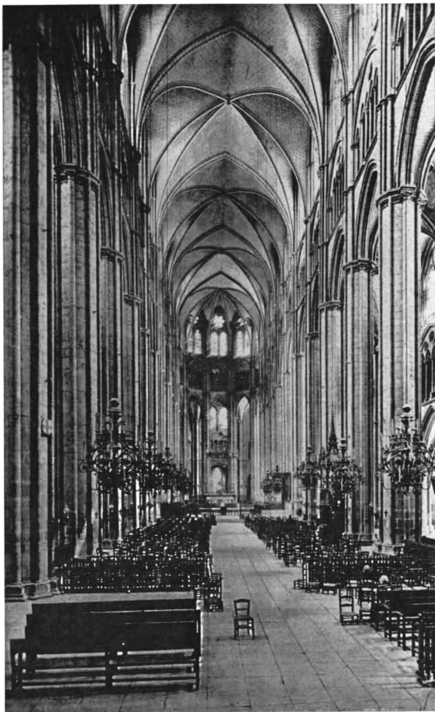
MAIN VAULTING of Bourges rises 120 feet above the floor. Whereas the vaulting of Chartres and almost all other High Gothic cathedrals is quadripartite (see illustration on page 92), Bourges's vaulting is sexpartite. Alternate piers meet one vault rib or three ribs.
