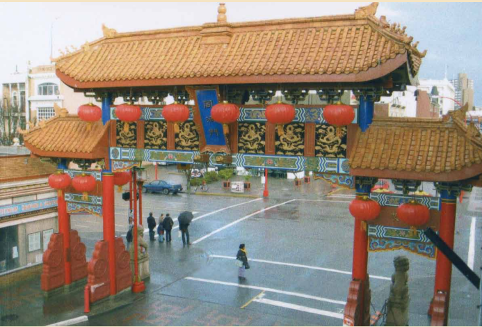
Erection of the Gate of Harmonious Interest “同濟門”牌樓
