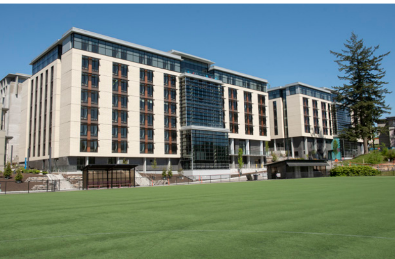
Phase 1 of our new student residence buildings
