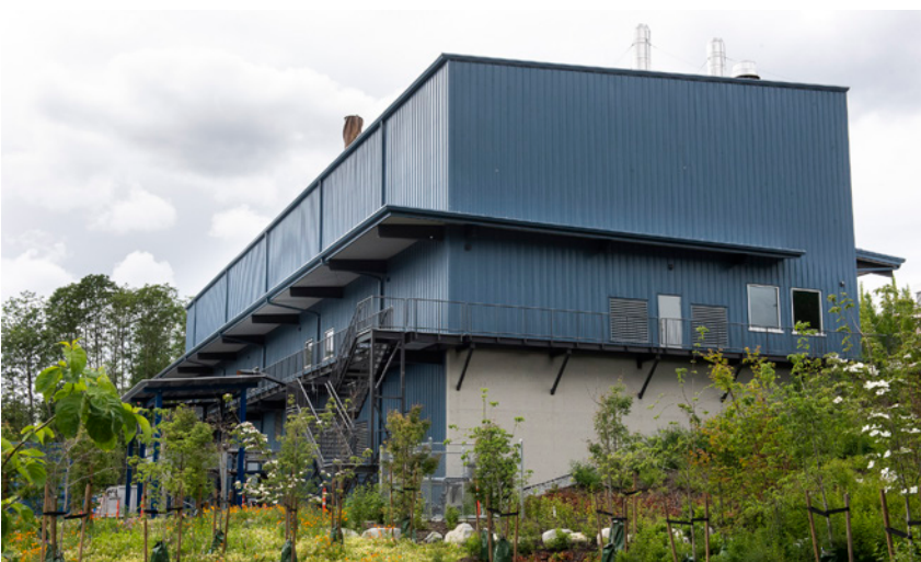
Corix biomass plant
