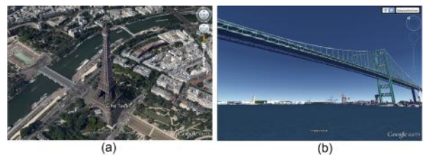
Figure 6: (a) The Eiffel tower in Paris. (b) The Vincent Thomas Bridge in Los Angeles. Images taken from Google Earth [5].
