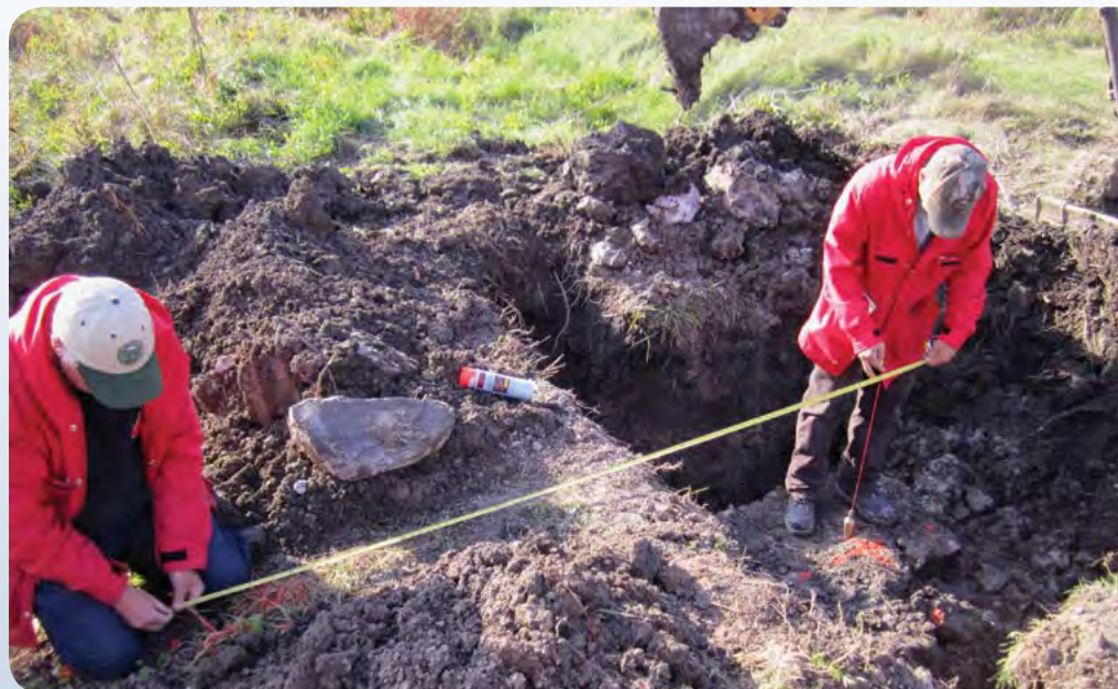
A crew works to locate an international boundary marker on the Quebec-Vermont border.
